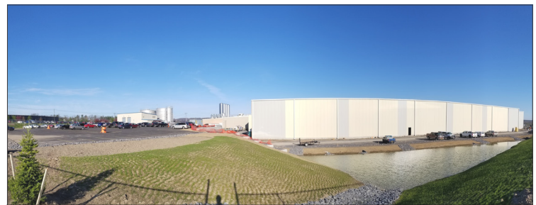
Construction inspection photo of KanPak, Penn Yan, NY
