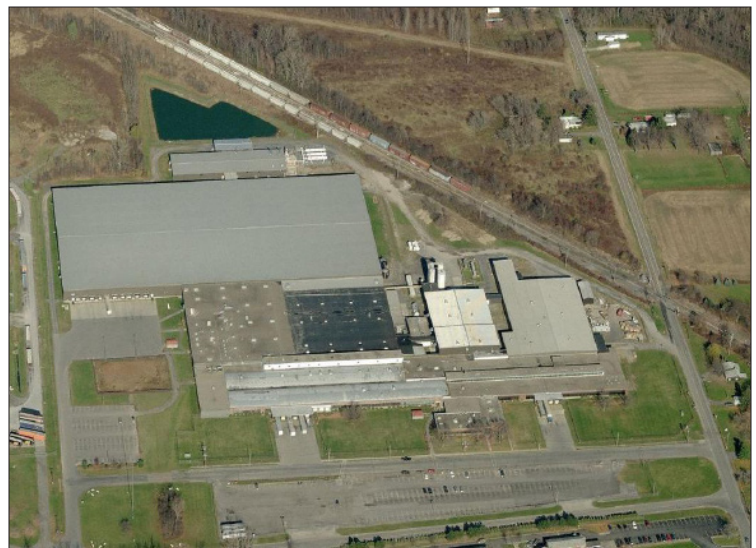
Aerial image of Zotos Warehouse, Geneva, NY
