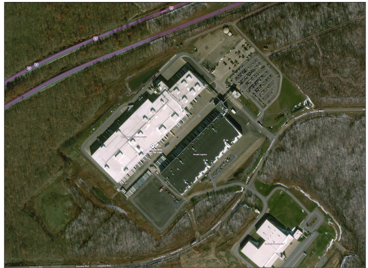
Aerial image of Wegmans Retail Service Center, Pottsville, PA
